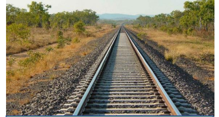
Ctg. - Cox's Bazar Rail Link Project
