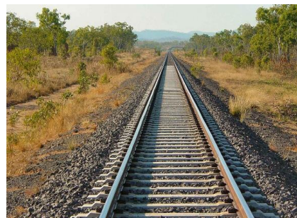
Ctg. - Cox's Bazar Rail Link Project
