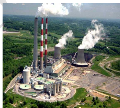
Matarbari Coal Power Plant
